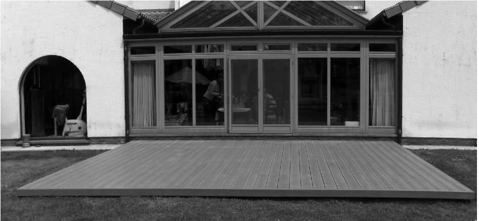
Rectangular decking with finishing border. The bearing structure is fixed to the wall.
