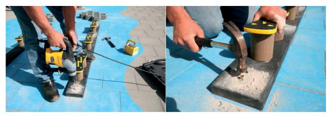
The elements have pre-drilled holes for anchoring. You only have to position the elements correctly and drill the holes with an 8 mm stone drill. Then secure with the 8x100 nail plugs. Advice: first place the plastic plug, then place the metal nail.
