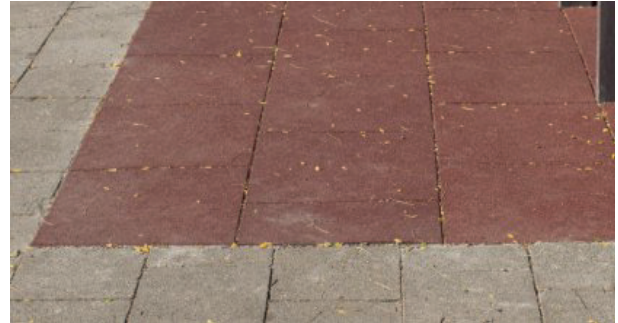
Rubber tiles sunk to the level of the surrounding paving. Better finishing but more work. (remove existing paving, and install a bed of stabilised sand or compacted stone chippings)
